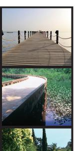
H6 - High Hazard: Prolonged immersion in sea water (Marine piling, jetty cross-bracing, landing steps, retaining walls etc.)
